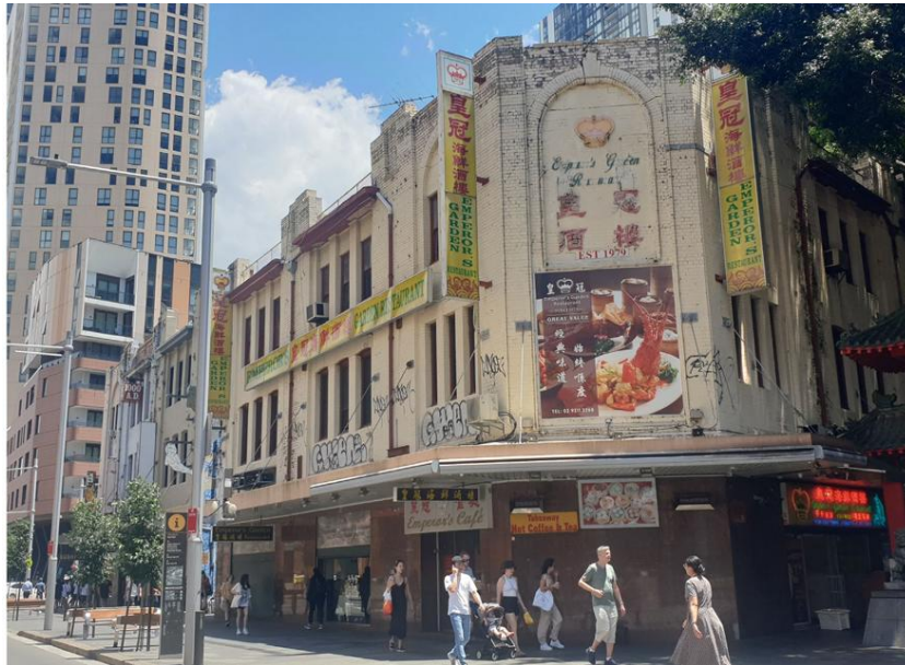
Figure 3 – View of Hay Street façade of subject site. (Source: City of Sydney)
