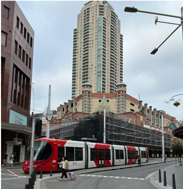
Figure 7 – Market City, opposite Hay Street to the south (Source: Planning Lab)
